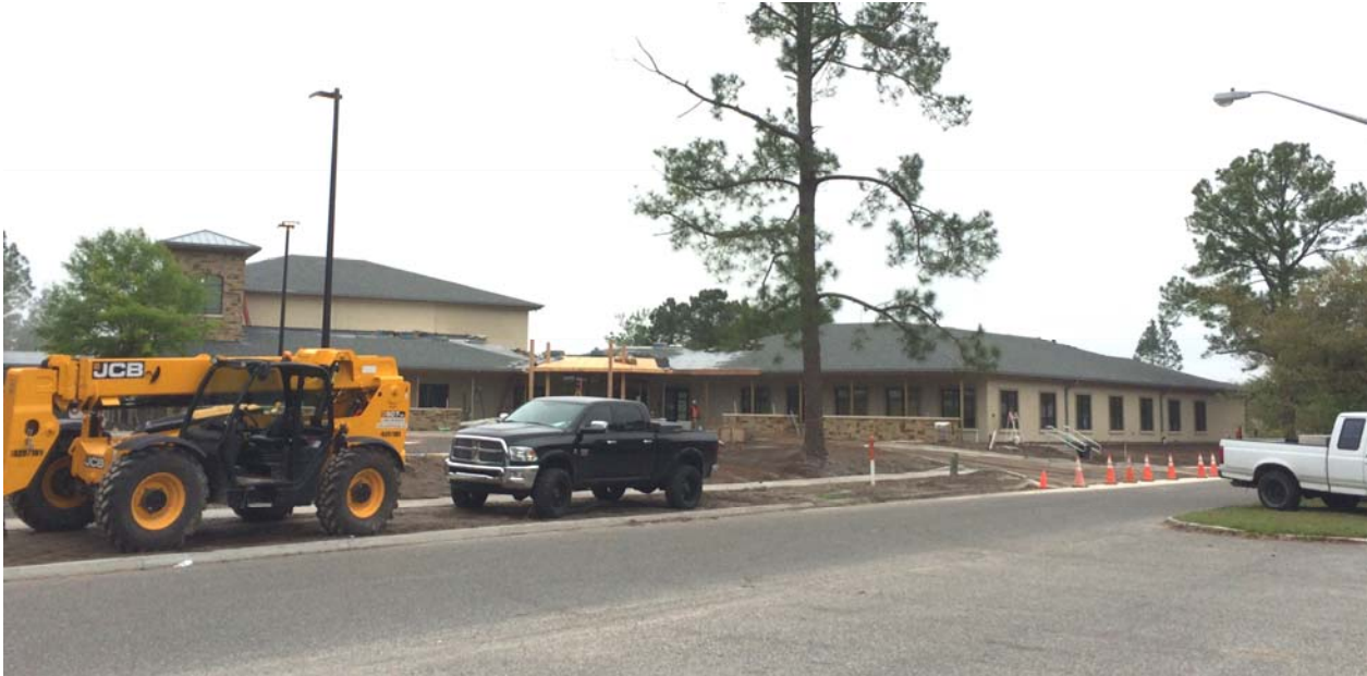
View of existing facility facing northwest
