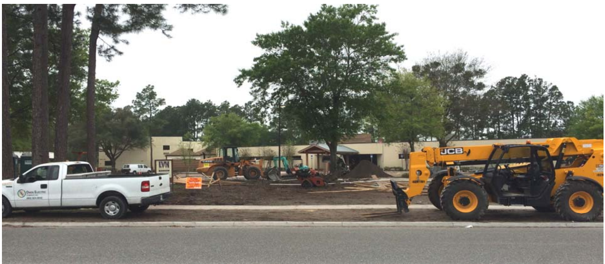
View of existing facility facing west
